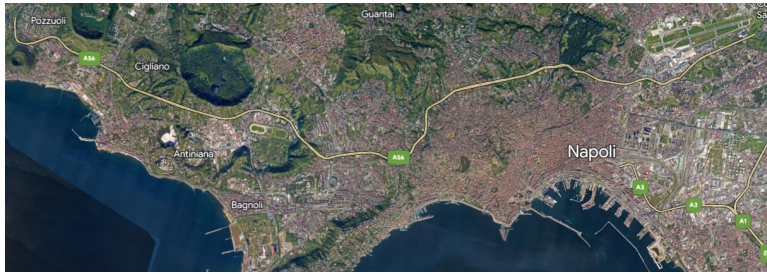
(a) Overview of the A56, highlighted in yellow.
